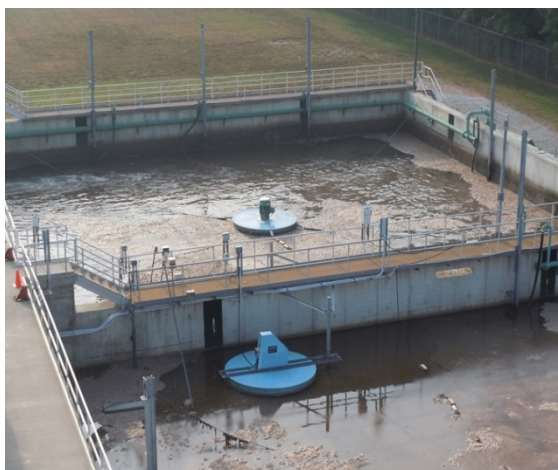
Figure 3: Sequencing Batch Reactors at Different Stages (Aqua-Aerobic Systems, Inc.)
