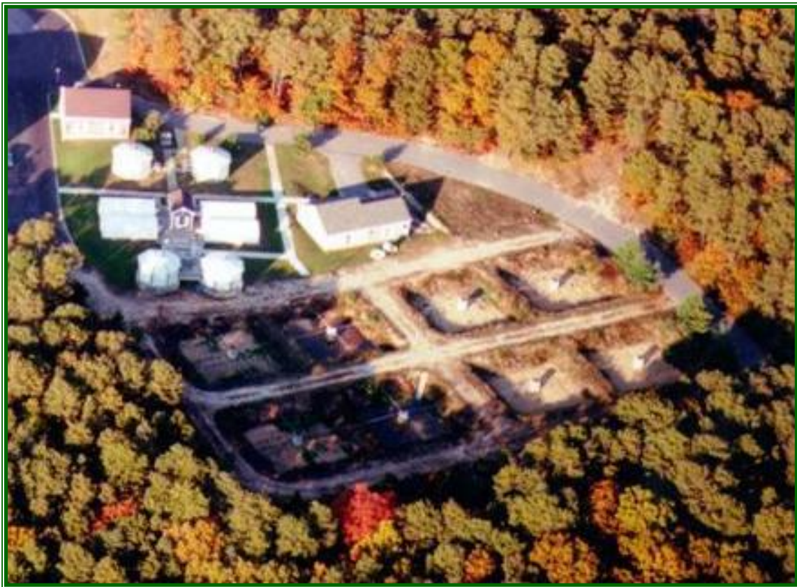
FIGURE 5-2 TRI-TOWN SEPTAGE TREATMENT FACILITY
