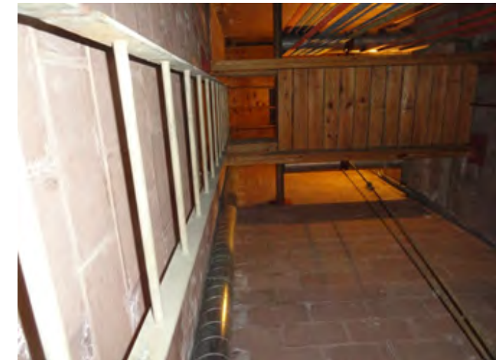
Photo #16 Hose Tower - interior masonry
