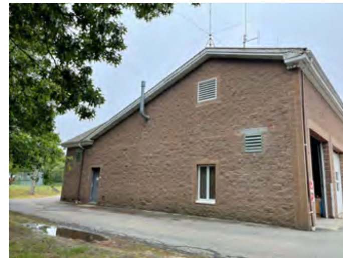
Photo #5 Building North Elevation
