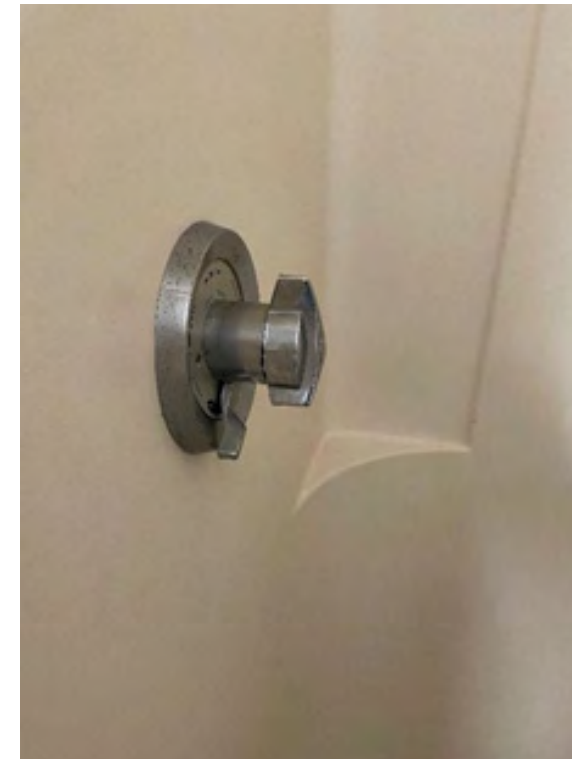
Existing Shower Valve
