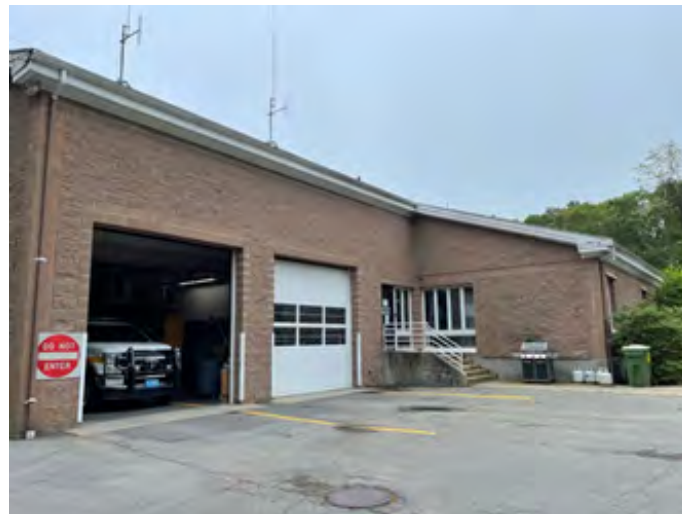
Photo #3 Building West Elevation Rescue Vehicle Garage Doors
