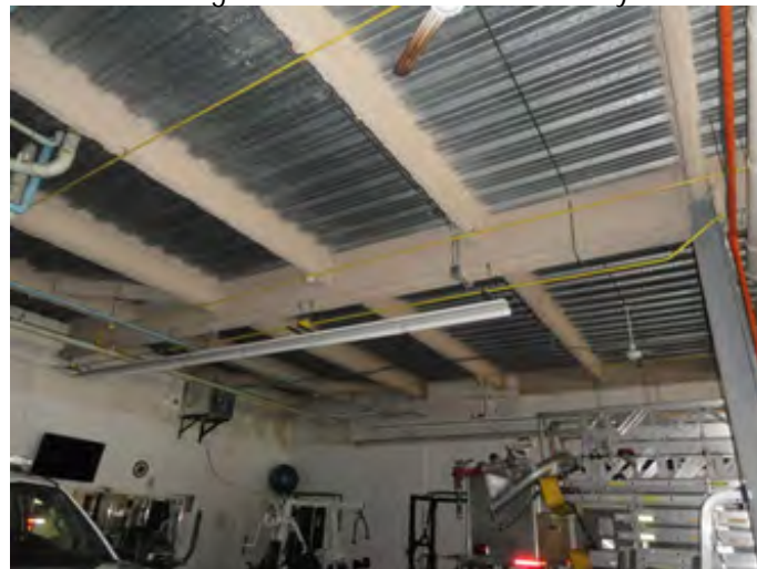
Photo #13 First floor steel framing above the main apparatus bays
