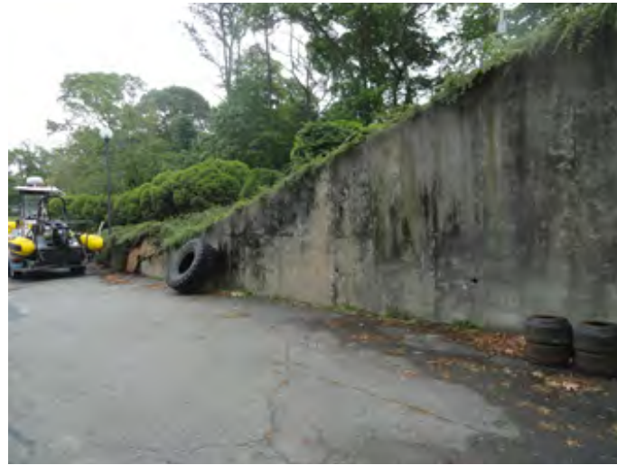
Photo #9 South Retaining Wall
