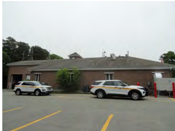
Photo #2 Building West Elevation
