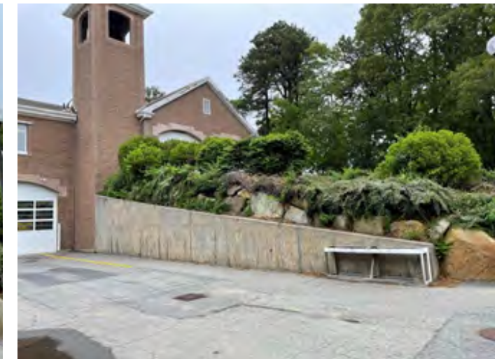
Photo #8 North Retaining Wall
