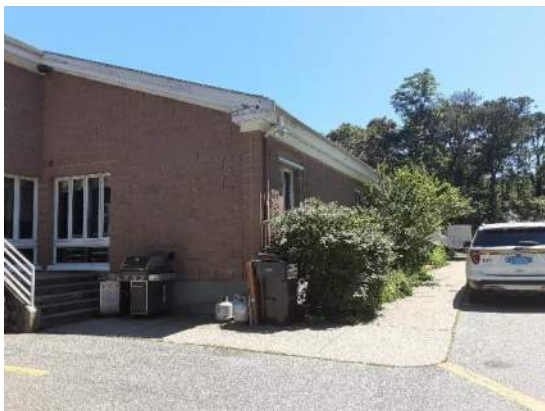
Figure 1.3. East face of building and staff entry
