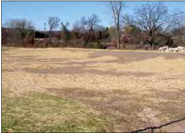
Figure 4h. Straw mulch needs to be held in place to prevent movement from wind especially if chopped. Photo by John Price, Price and Company.
