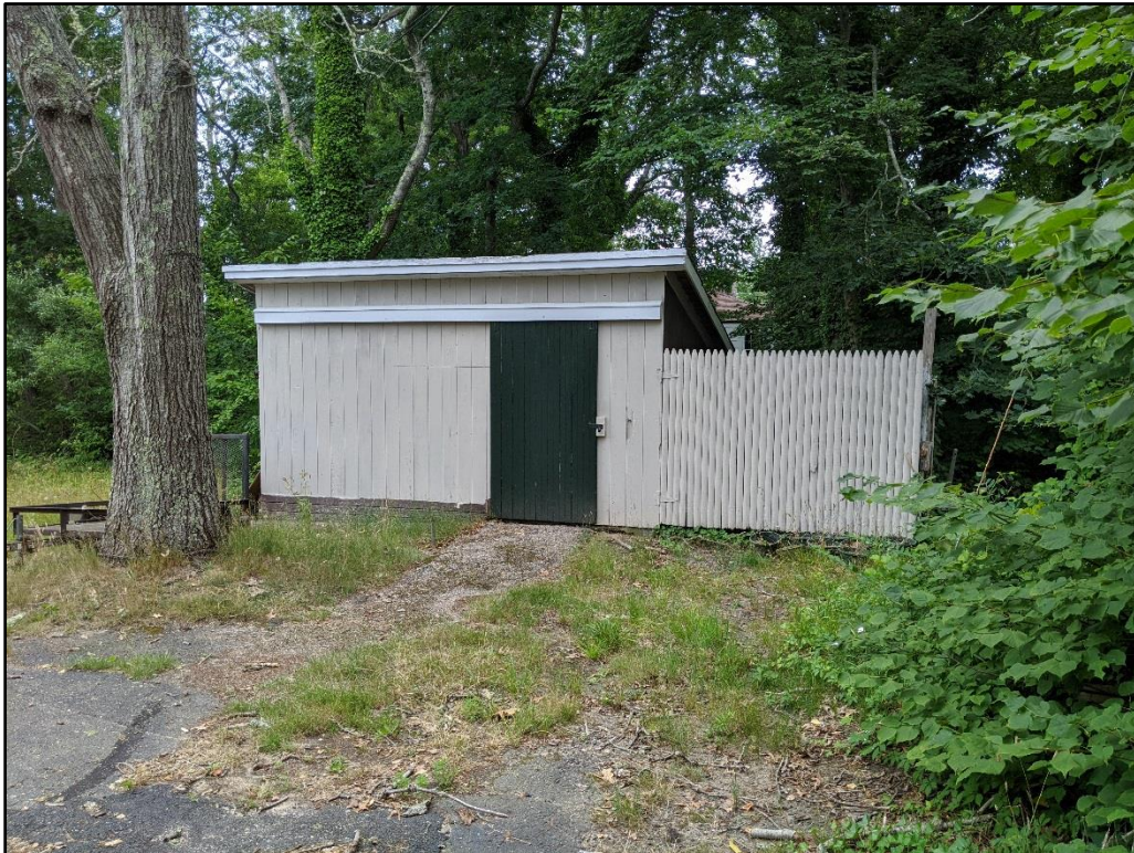
Tractor Shed, located southwest of the Main Building.
