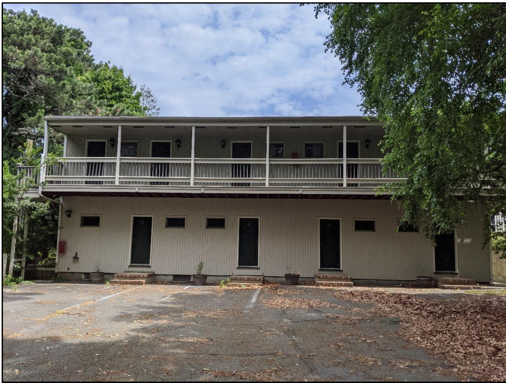
Rear of Pool Building, view facing east.
