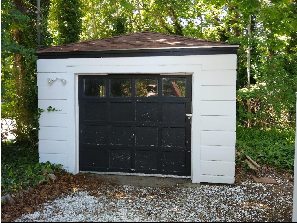
Detached garage off of the building at 76 Rt 6A property.
