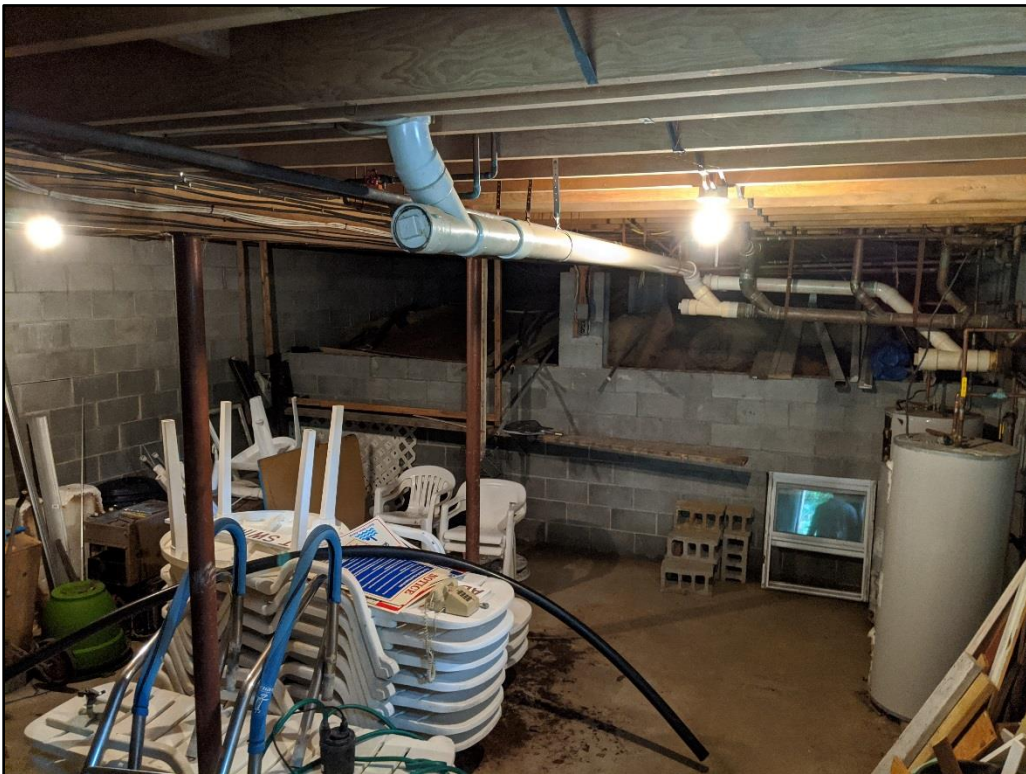
Pool Building basement.
