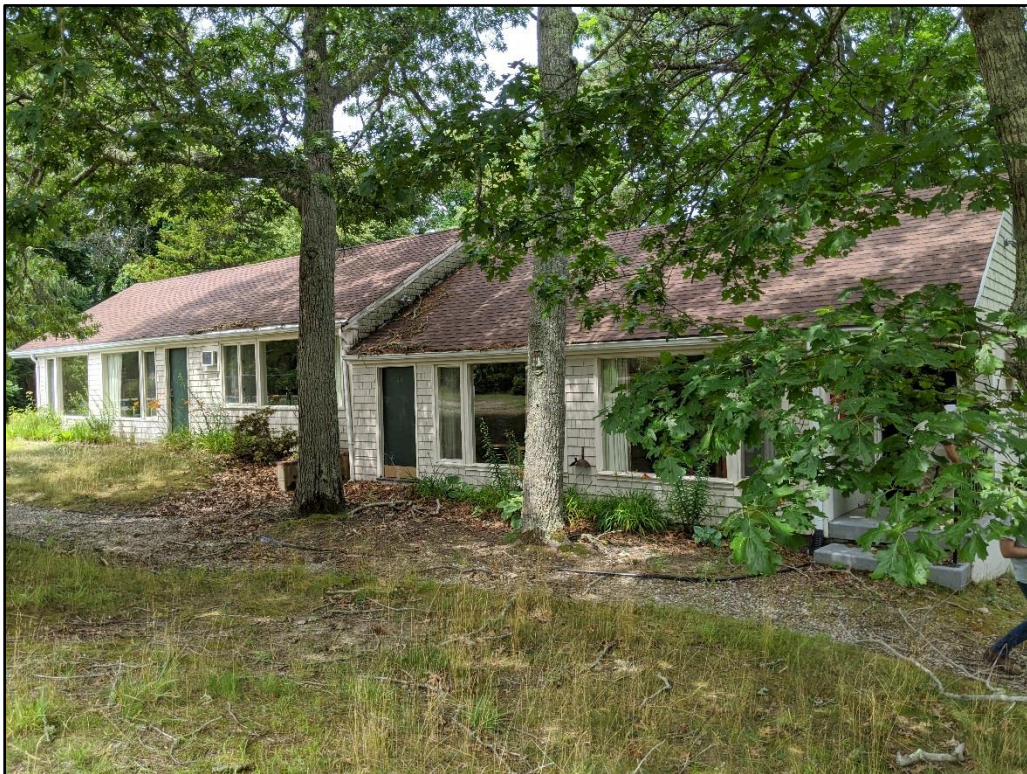
Courtyard 2 building, view facing northwest.
