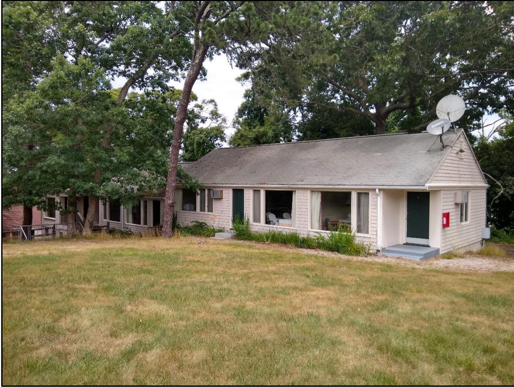
Courtyard 1 building, view facing northeast.
