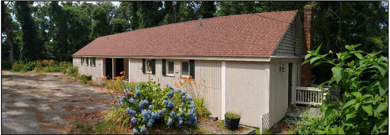
Woods View building, view facing North.
