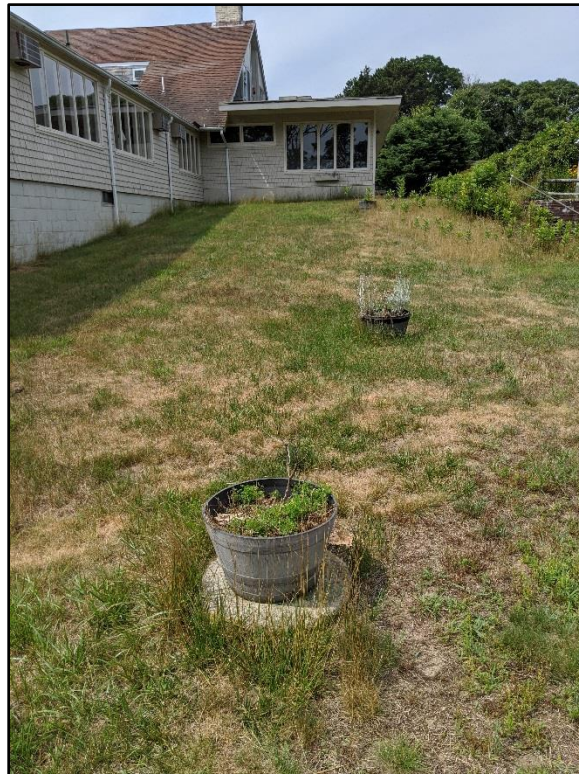
Rear of main motel building, view facing southwest. Concrete covers mark locations of former cesspools.
