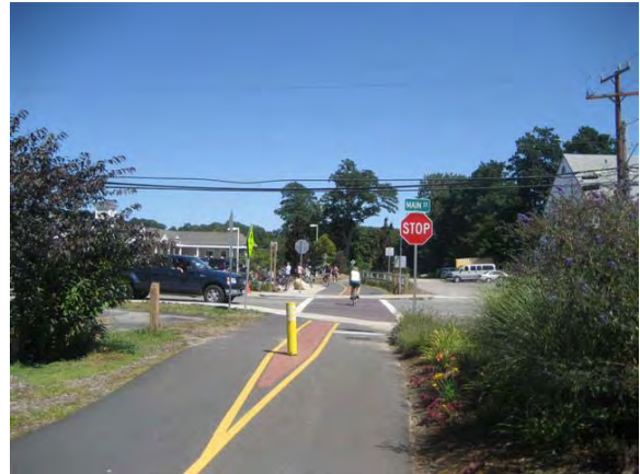
Figure 1: Cape Cod Rail Trail Main Street Crossing
