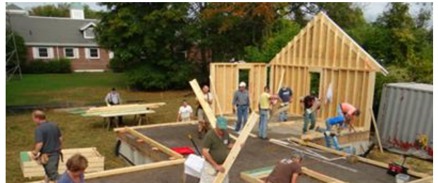
Habitat for Humanity Project
