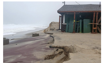
Liam’s Snack Shack Demolition, 2018
